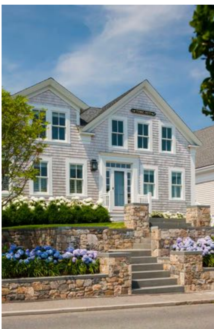
The home's Greek Revival style is important to a Chatham village steeped in history. The renovation restored historic architectural elements to the house's front and removed a series of telescoping rear additions, replacing them with a two-story ell. BRIAN VANDEN BRINK/POLHEMUS SAVERY DASILVA ARCHITECTS BUILDERS
